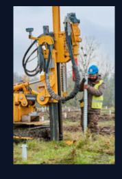
Suitable for all terrains, ground screws can be used in all soil types, including rock. When pre-drilling is required, no additional concrete or material is needed in the soil. No resting time is required, and the structure can be erected immediately.
