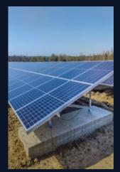
This unique solution is ideal for situations where screw or pile foundations are not possible, such as when there is a waterproof membrane (landfills). Offering exceptional adaptability to terrain leveling defects, it allows the structure to evolve with topographical changes (differential settlement). It also provides a solution for specific constraints, such as the presence of underground infrastructure.
